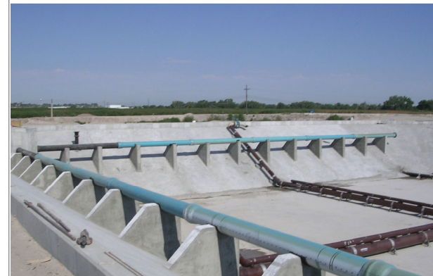
Waste Water Treatment Plant Aeration Basin
