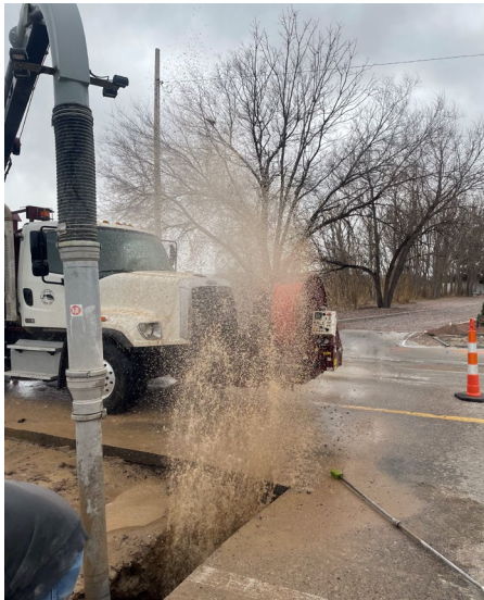
Water main repair
