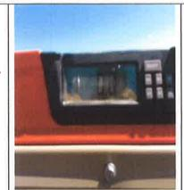
Units are not level will cause water from the condensate to leak inside od building
