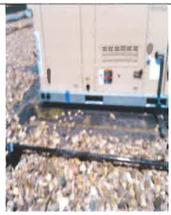
Units are not level will cause water from the condensate to leak inside od building
