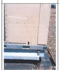
There are no ptraps on all units causing water to leak inside the building
