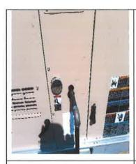
Gas piping missed the knock out so drill a new hole Missing rubber grommet causing water to enter the unit on all units
