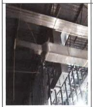
Strapping not to code with the use of plumber strap should be with Unistrut and allthread or at the minimum of a 1"20 gauge strap with a sheet metal cee channel
