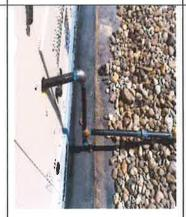
Improper attaching of exhaust piping there should be a appliance connection from single wall to double wall pipe
