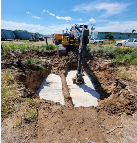
Water main repair on I Street
