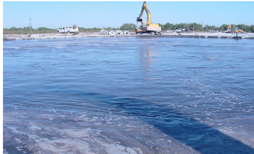
Wastewater Pond on U Street
